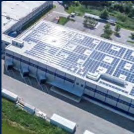
Solar panels in our plant in Memmingen, GER
